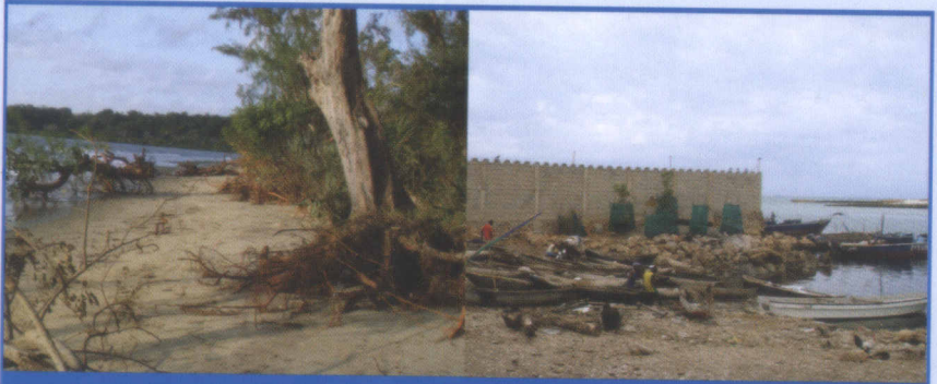
Beach erosion in Pangani (left), erosion threatened structures at Kunduchi - Dar es Salaam (right)
