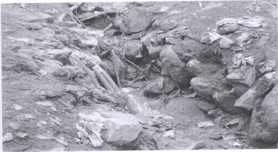
Plate 2: A wastewater open channel in Tandale informal settlement. Wastewater from the pit latrines been channeled into this local drainage system. The channeling of households' liquid waste into local drainage systems has been the source of surface and underground water pollutions. The people living in the area are susceptible to cholera and typhoid diseases (Photo: Hambati, 2014).
