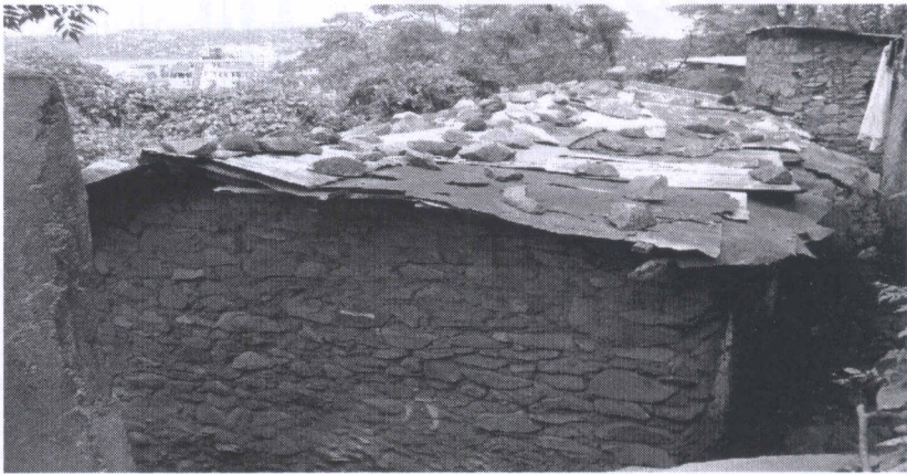
Photo 1: House made of low quality materials in Pamba informal settlement (Photo: Hambati, 2011).
