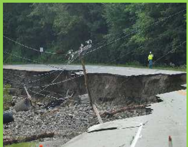
Damaged road infrastructure due to floods along Makuyuni - Karatu Road in 2011
