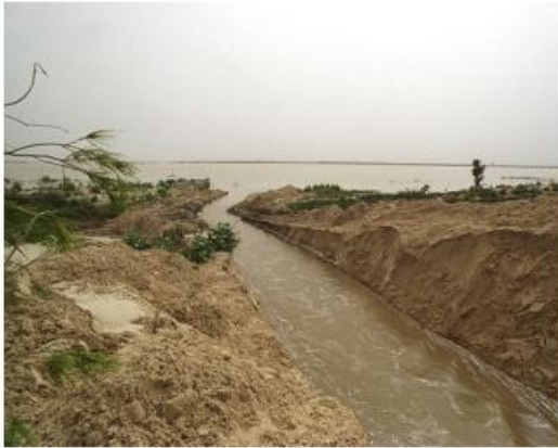
A) just after the opening of the breach, 3rd Oct 2003: 4 m width
